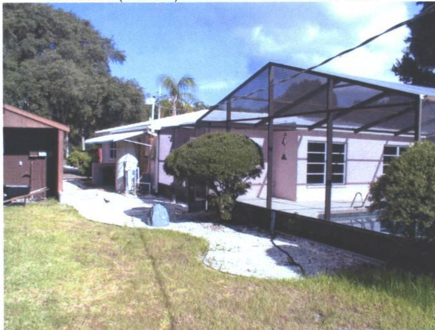
FIGURE 4: (06/22/11) RIGHT SIDE VIEW FROM REAR
