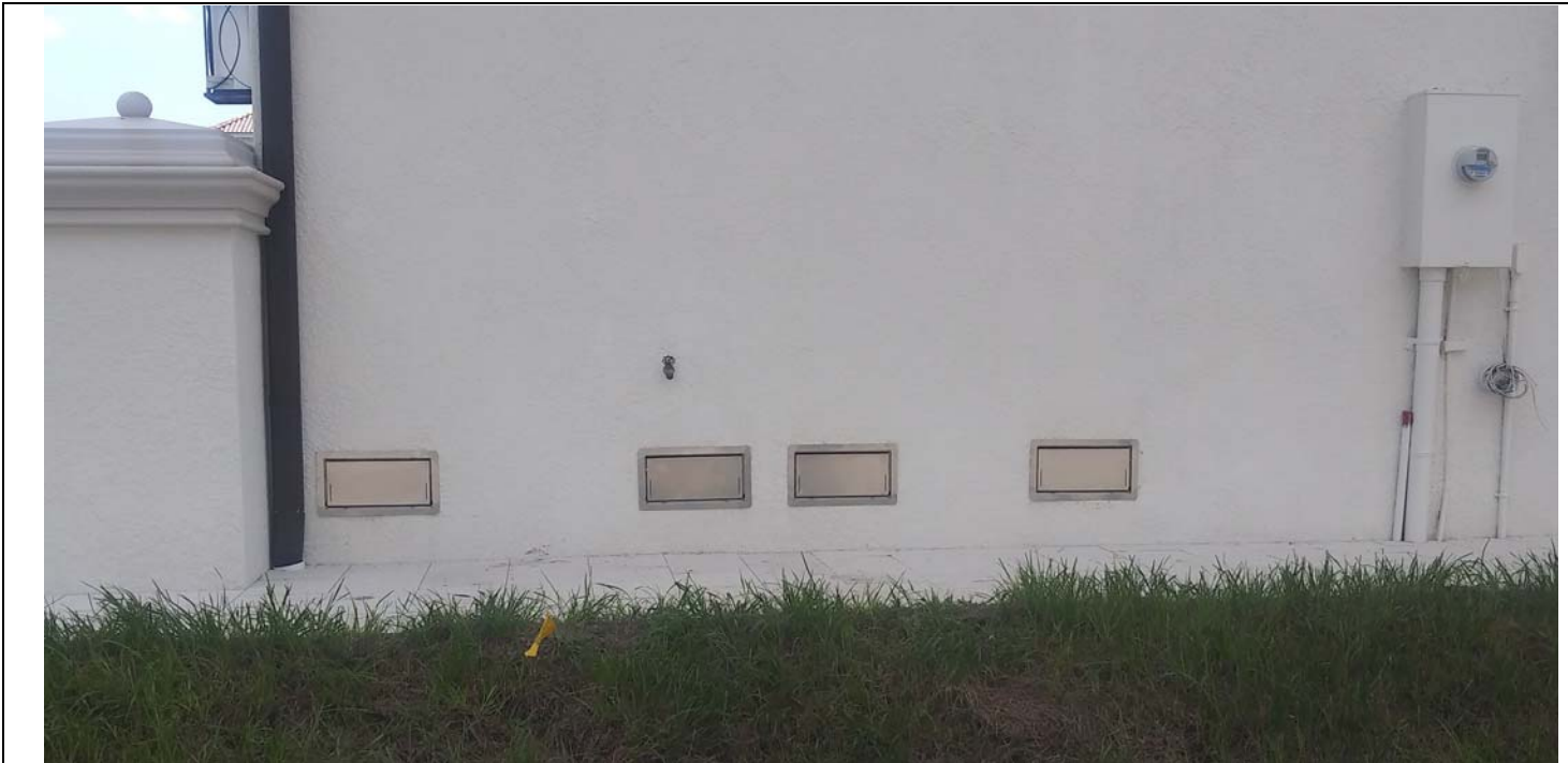
Photo 5 Caption Garage wall Flood vents JOB# 18-1123 Date Taken 10/13/20
