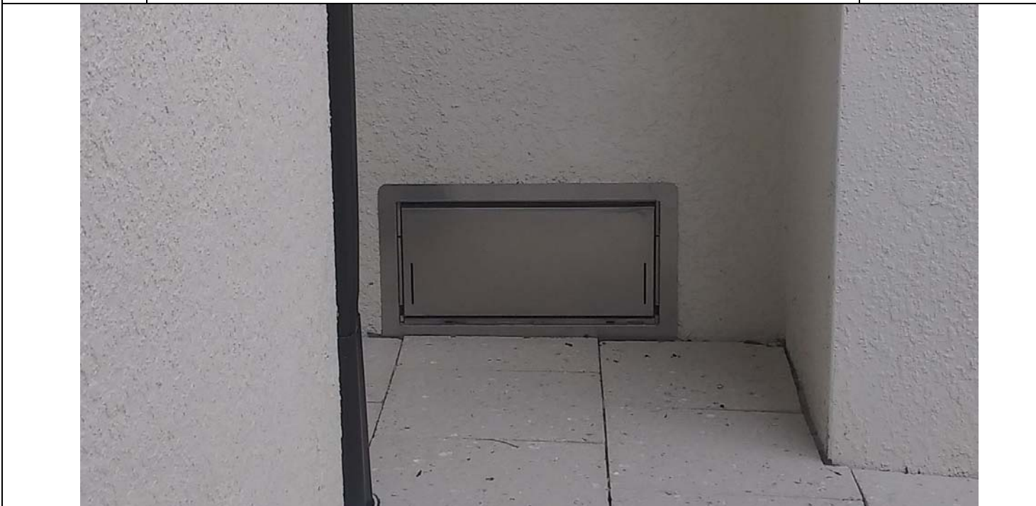
Photo 6 Caption (Typ) Garage wall Flood Vent JOB# 18-1123 Date Taken 10/13/20
