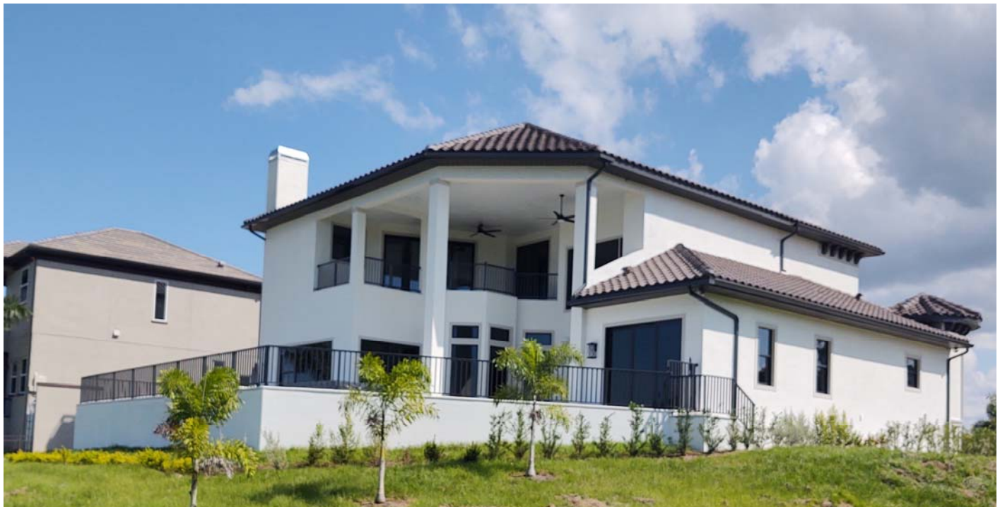
Photo 2 Caption Rear View JOB# 18-1123 Date Taken 10/13/20
