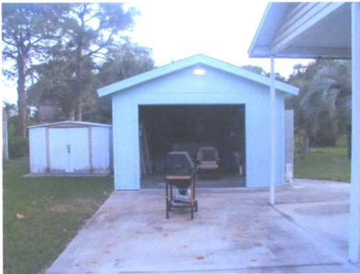
FIGURE 5: (11/06/13) FRONT VIEW DETACHED STRUCTURE
