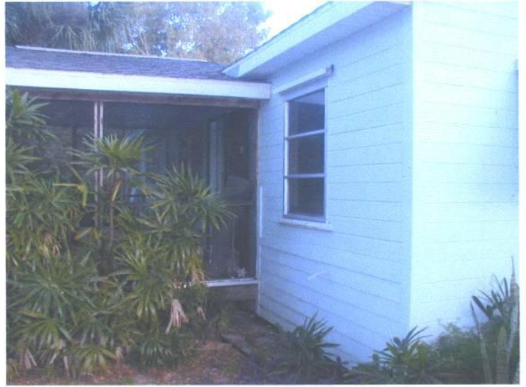
FIGURE 2: (11/06/13) FRONT VIEW FROM RIGHT SIDE (SCREENED PORCH/ENTRY)
