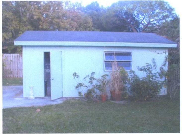
FIGURE 6: (11/06/13) RIGHT SIDE VIEW DETACHED STRUCTURE
