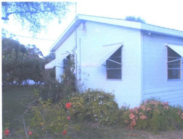
FIGURE 2: (11/06/13) RIGHT SIDE VIEW FROM REAR
