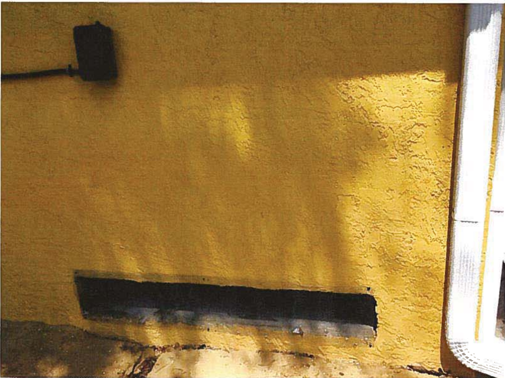
Styrofoam removed from flow through openings.
