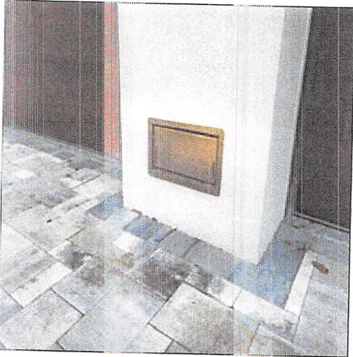
VENT PHOTO TAKEN ON DECEMBER 11 2024
