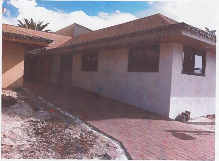
NW Corner - window sills above base flood elevation
