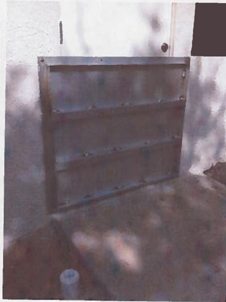
Rear Door Flood Panel Installation
