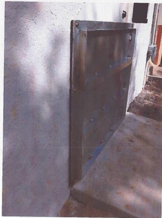
Rear Dr Flood Panel Edge Connection
