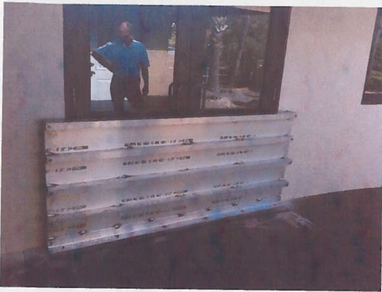
Front Door Flood Panel Installation
