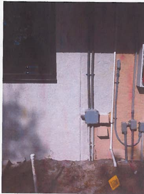
Expansion joint between new floodproofed structure and existing structure
