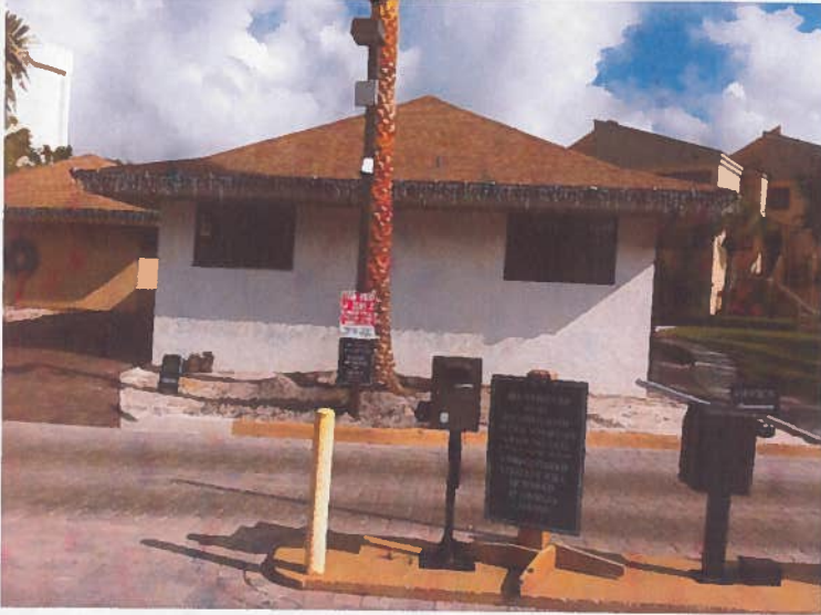
West Side - window sills above base flood elevation
