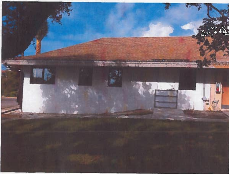
South Side - window sills above base flood elevation
