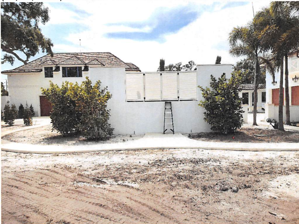
(04/24/2024) Detached Elevated AC & Generator Enclosed Platform =11.1'
