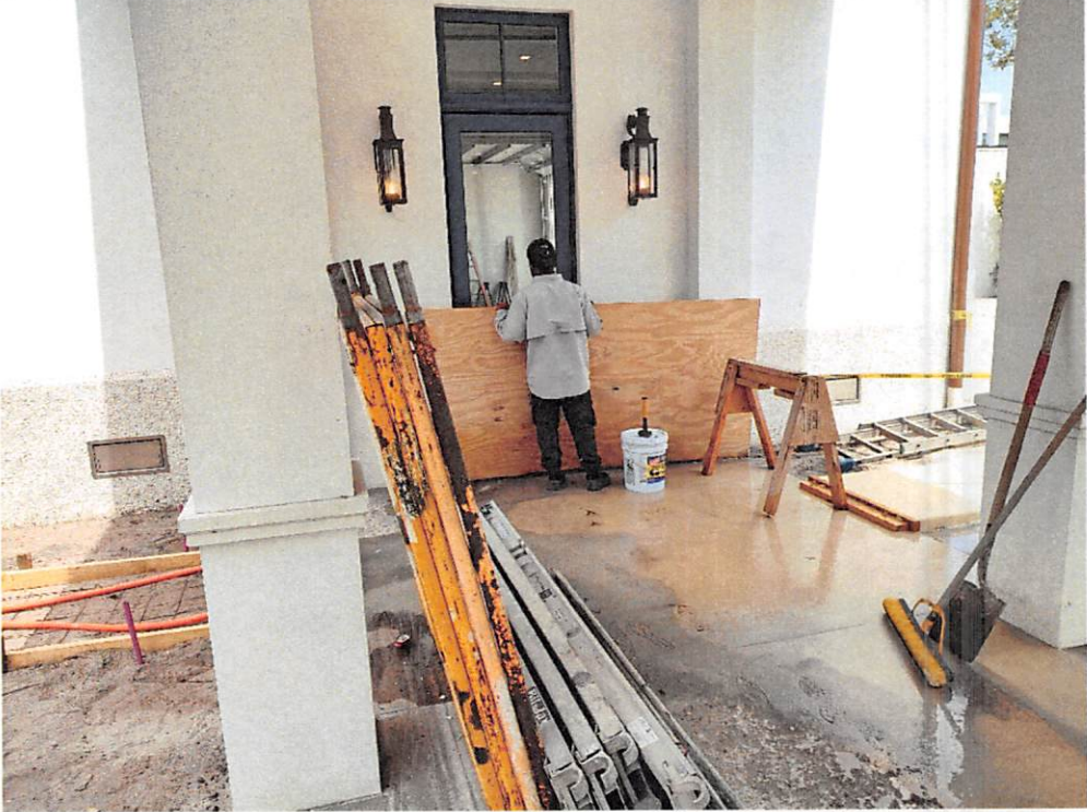
(04/24/2024) West Garage Wall with 2 Engineered Smart Vents.
