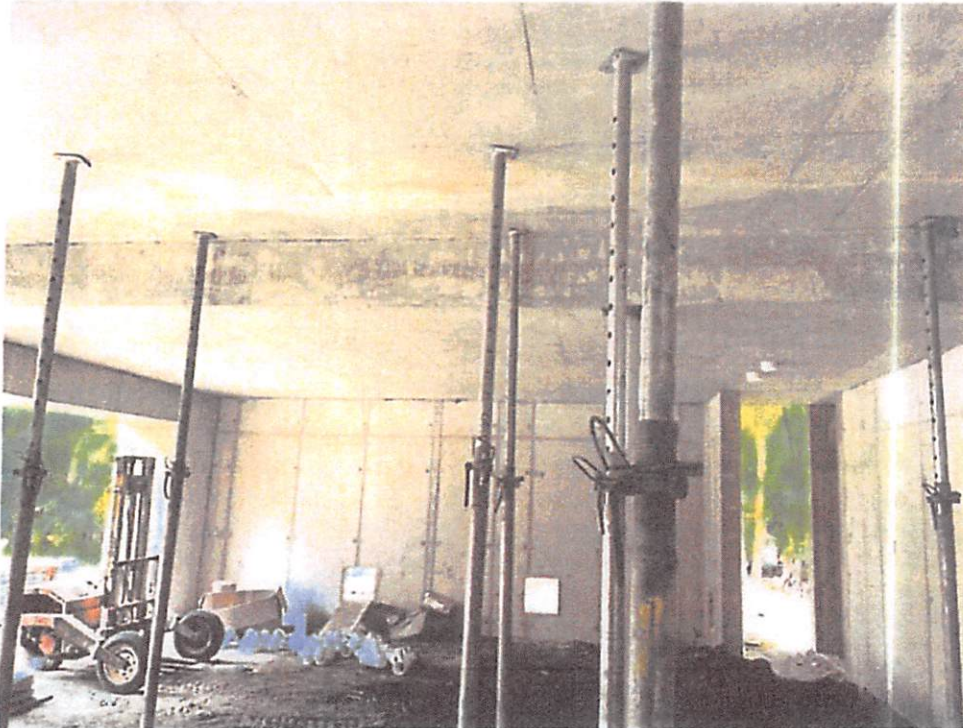
(02/22/2022) Lowest Horizontal Structural Member and Typical Flood Openings
