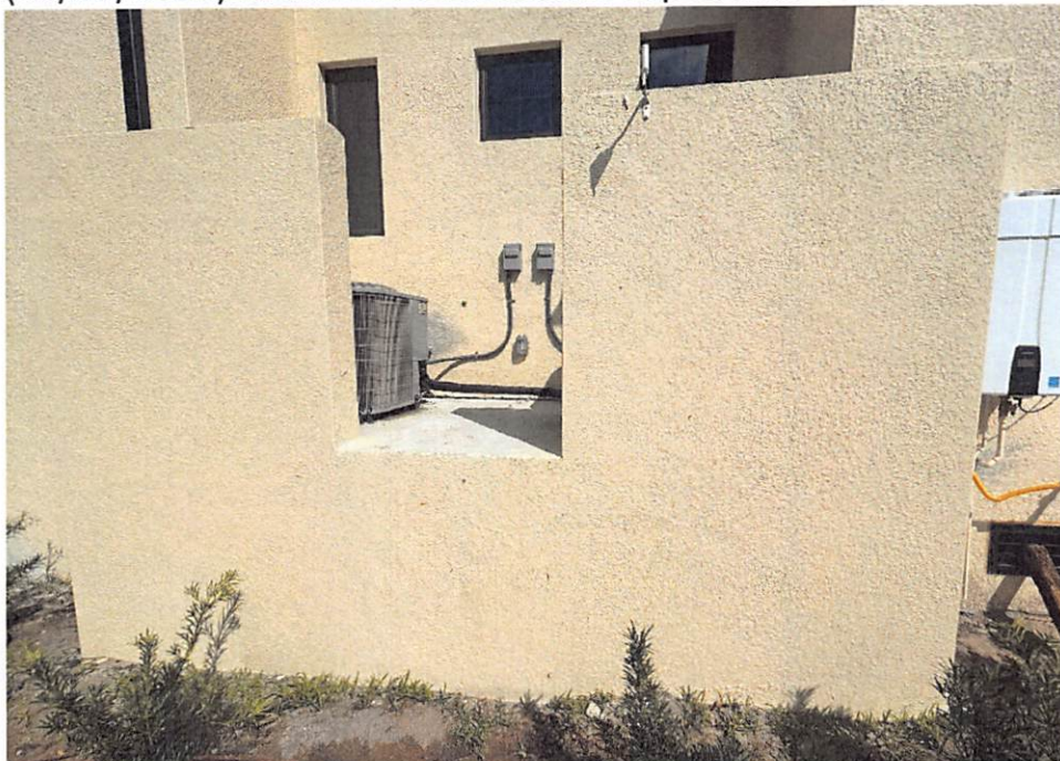
(05/27/2025) Elevated AC Enclosure Top of Slab=11.1'
