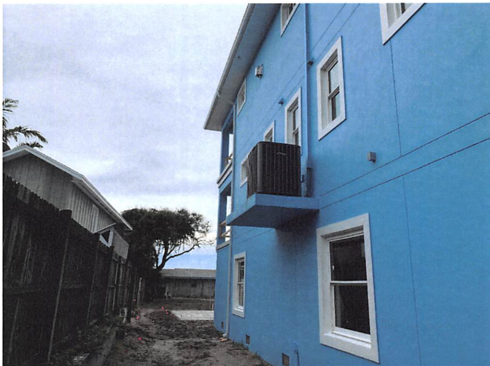
(08/19/2020) Typical Elevated AC and Exterior Flood Vents
