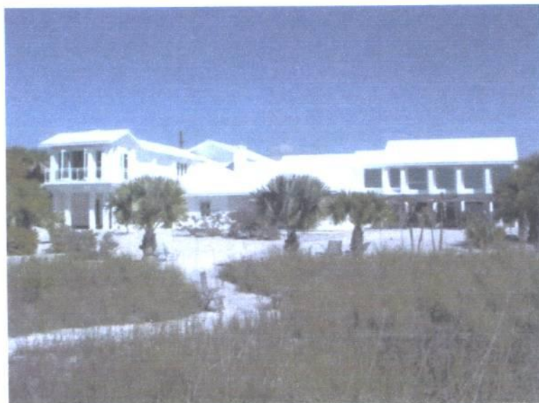
REAR VIEW OF NEW ADDITION (LEFT) AT 728 N. MANASOTA KEY ROAD, ENGLEWOOD, FL 34223
