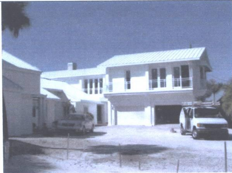
FRONT VIEW OF NEW ADDITION AT 728 N. MANASOTA KEY ROAD, ENGLEWOOD, FL 34223
