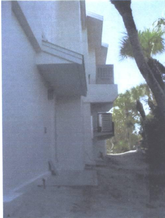
SIDE VIEW OF NEW ADDITION AT 728 N. MANASOTA KEY ROAD, ENGLEWOOD, FL 34223
