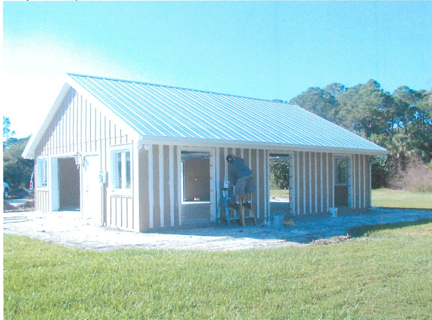
FIGURE 1: (10/28/13) FRONT & RIGHT SIDE VIEW SHOWING 3 FRAMED OUT FLOW THRUS
