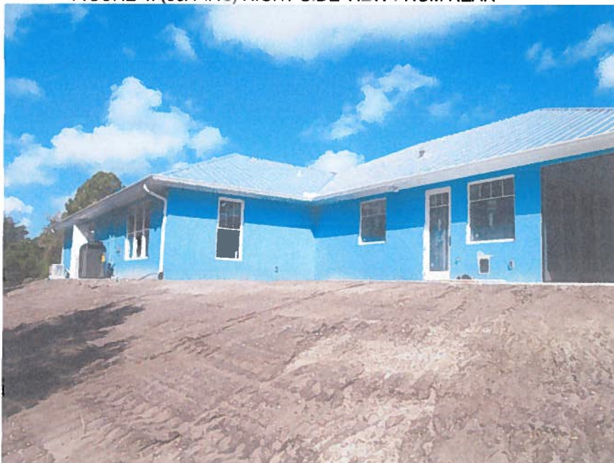
FIGURE 4: (05/14/15) RIGHT SIDE VIEW FROM REAR
