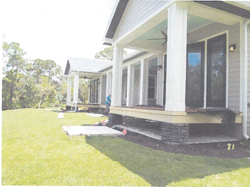
FIGURE 3: (09/02/14) REAR VIEW OF HOUSE FROM LEFT SIDE
