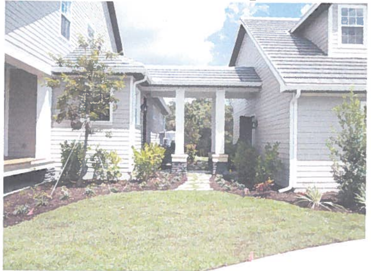
FIGURE 5: (09/02/14) FRONT VIEW BETWEEN HOUSE AND GARAGE
