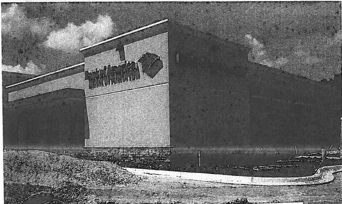
SOUTH AND EAST FACE OF BUILDING
