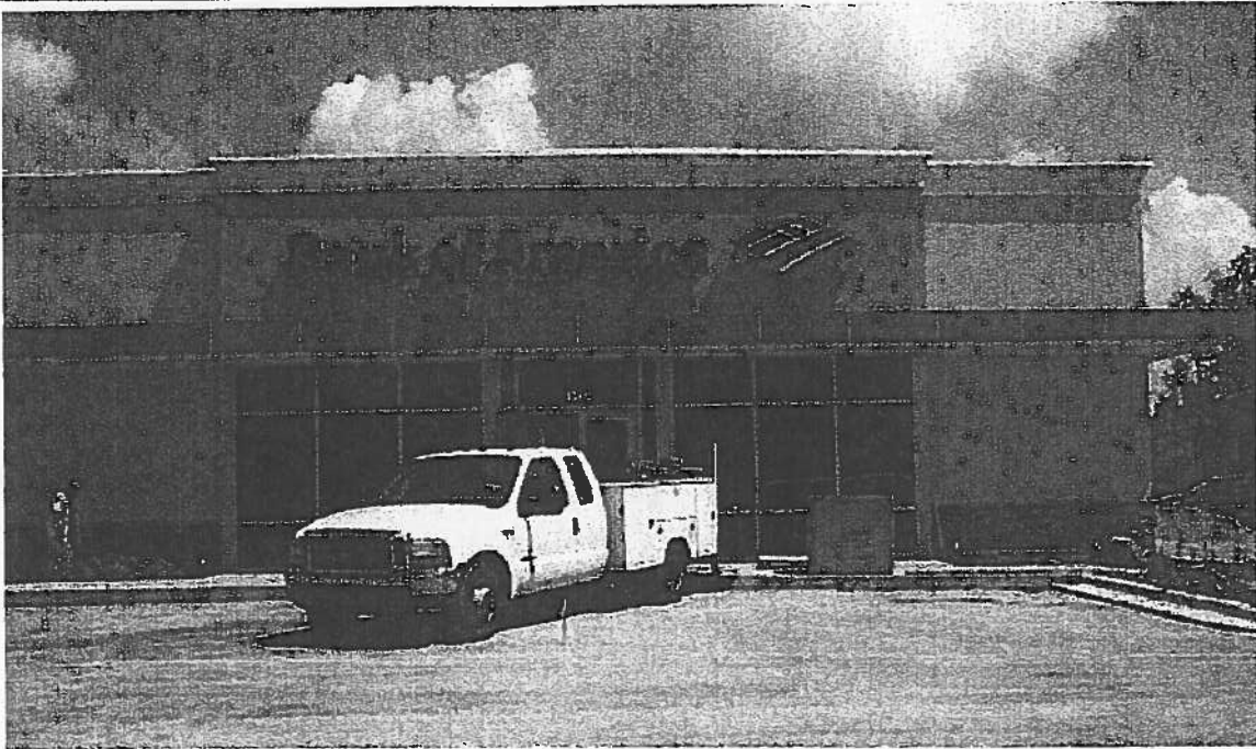
WEST FACE OF BUILDING
