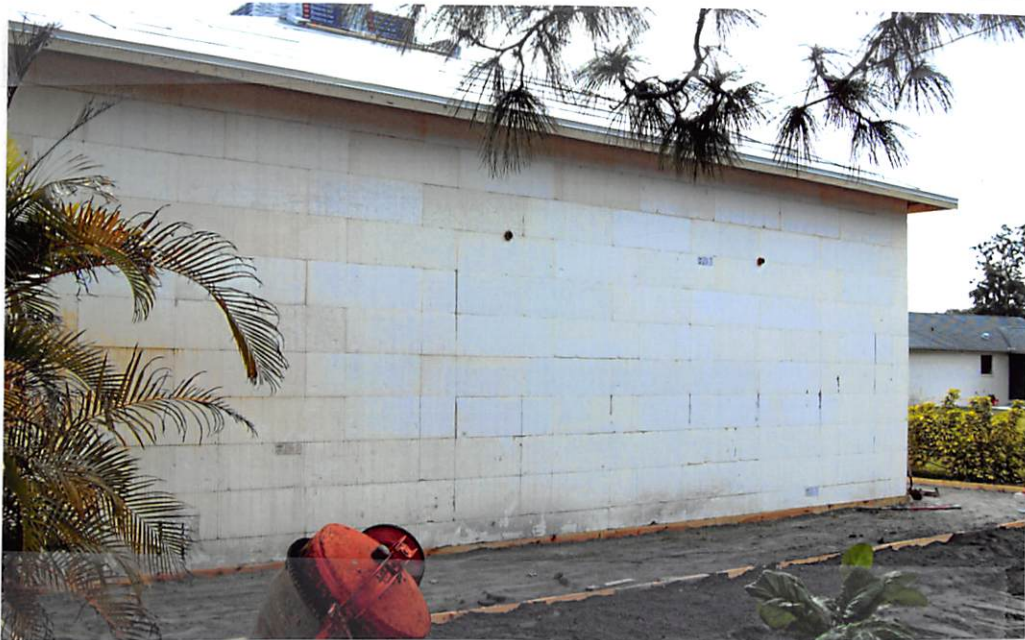
REAR (WEST SIDE)
