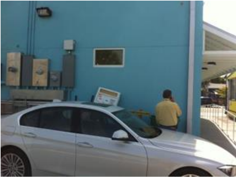
West Side – no openings below base flood elevation
