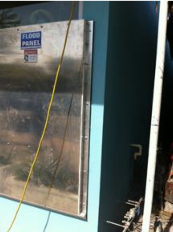
Typical Flood Panel Edge Connection
