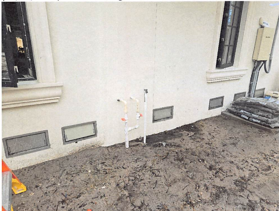
(10/01/2024) Portion of Right Side Wall at Rear, 6 Smart Vents
