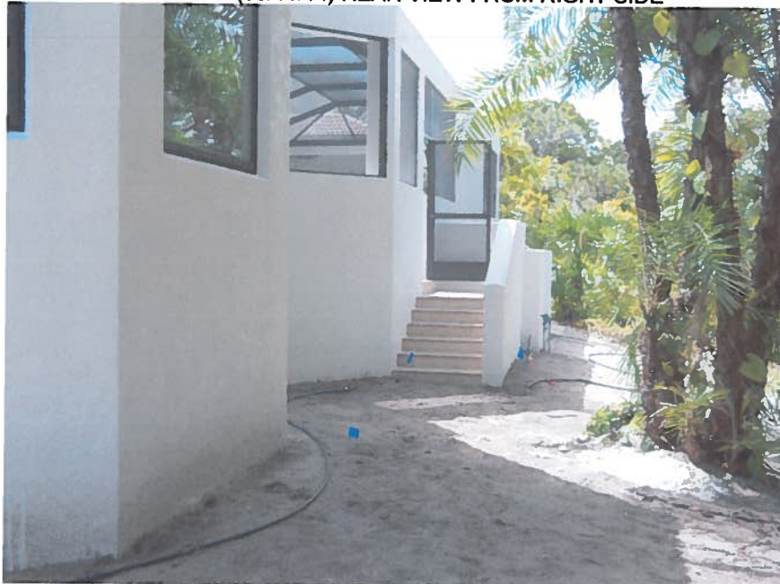
FIGURE 4: (08/11/14) REAR VIEW FROM RIGHT SIDE
