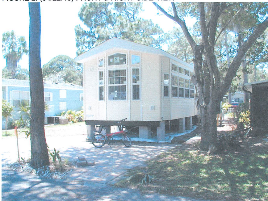
FIGURE 2: (04/22/13) FRONT & RIGHT SIDE VIEW
