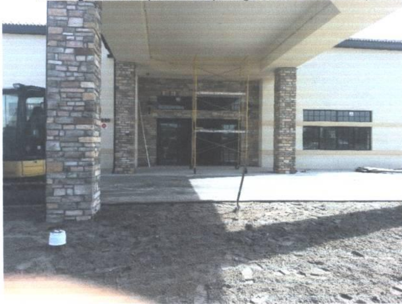
Building Entrance (Front view) image taken 11/19/2013)
