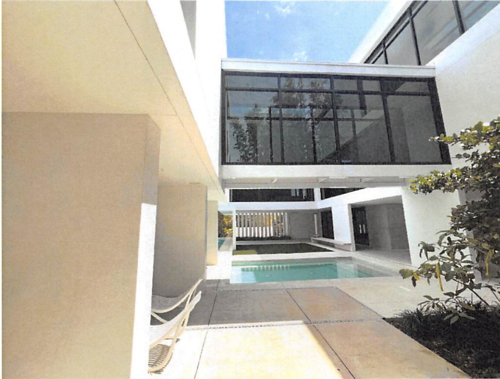
(04/18/2024) North Side of Addition with Connecting Walkover
