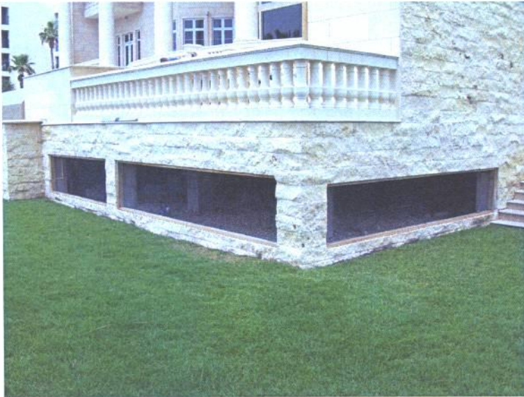
Rear View- Venting - 05.19.10
