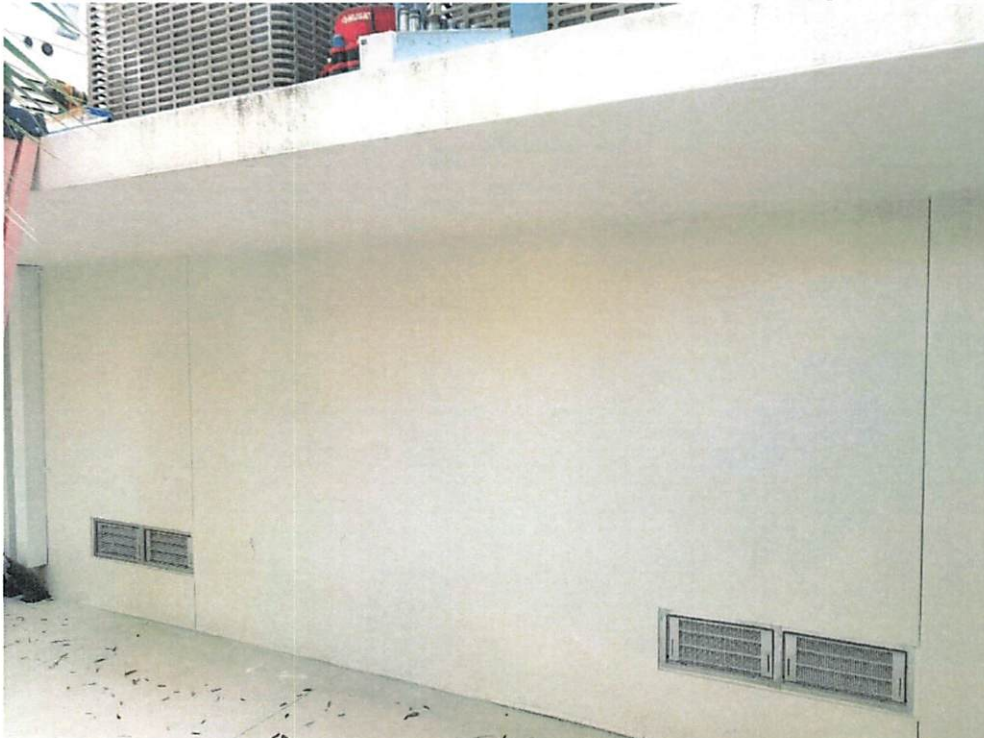
(12/21/2023) 4 Smart Vents Model #1540-510 in Garage 2, Left Side Wall Only
