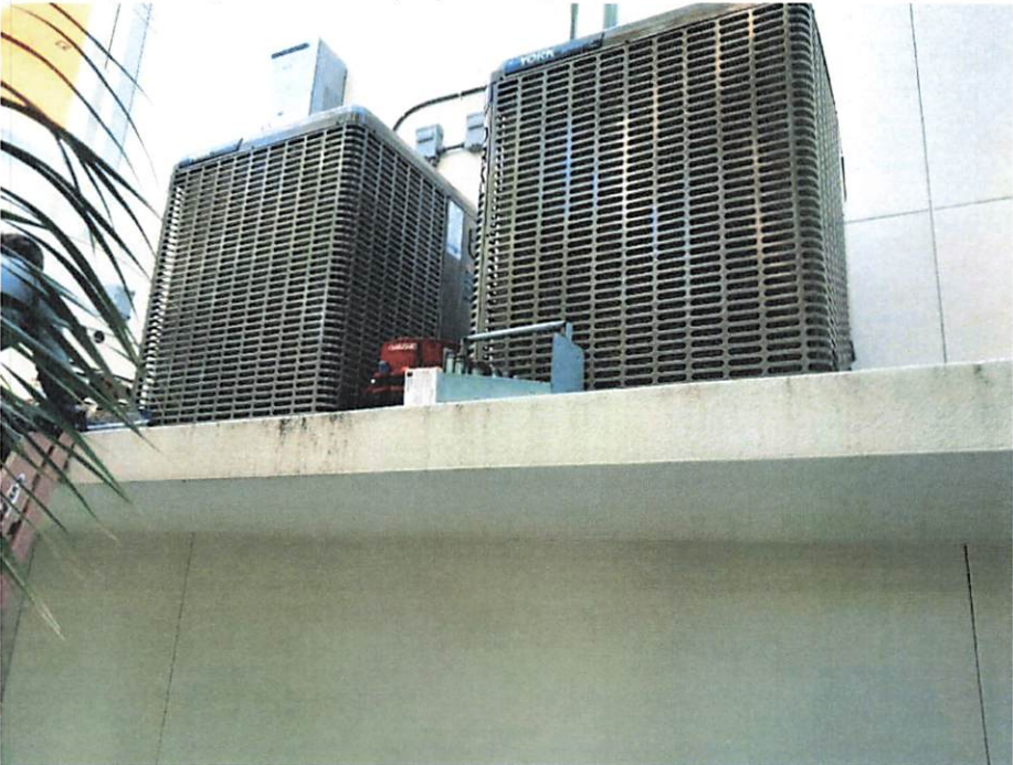
(12/21/2023) Lowest Equipment, Elevated AC Units = 12.0'
