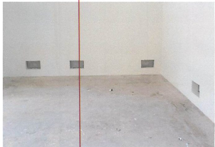
REPRESENTATIVE EXAMPLES OF FLOOD VENTS
