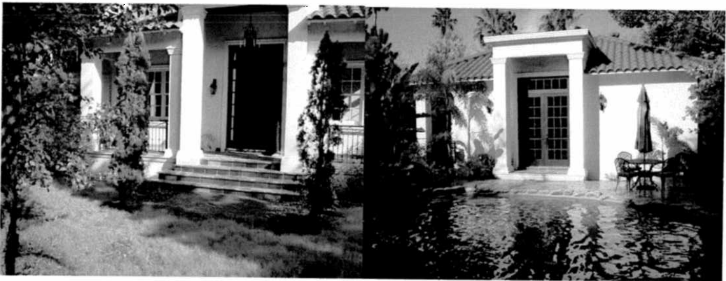
South Side - Toward Front of Building 3/07/10
