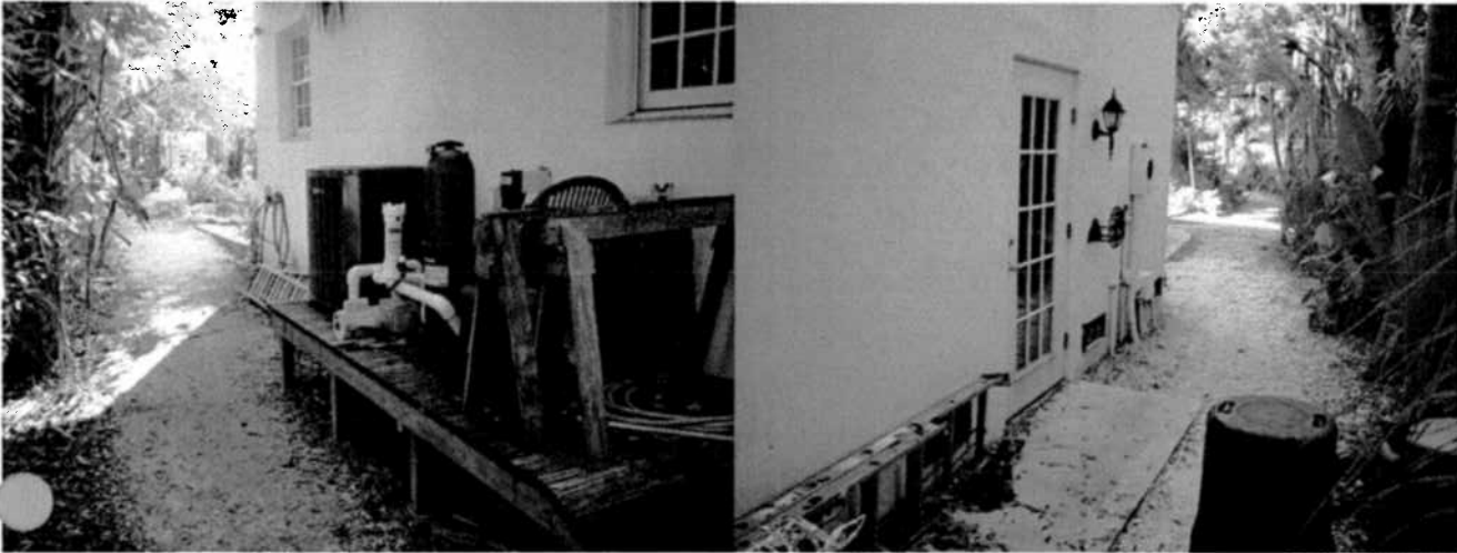
North Side – Looking Toward Front 3/07/10
