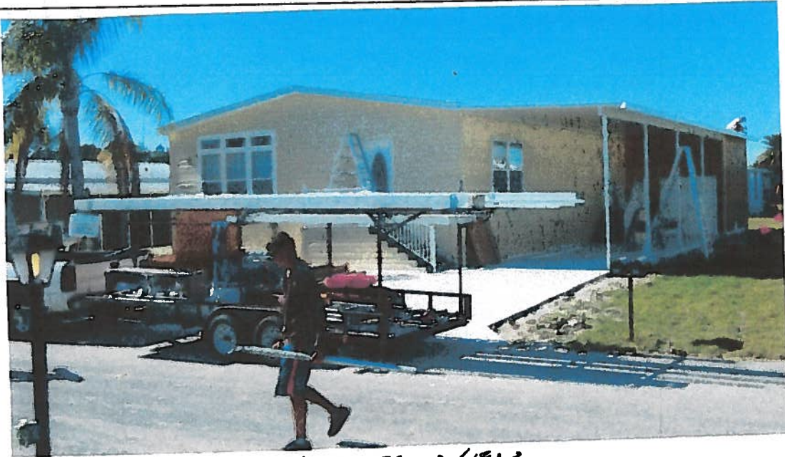
NORTH SIDE VIEW
