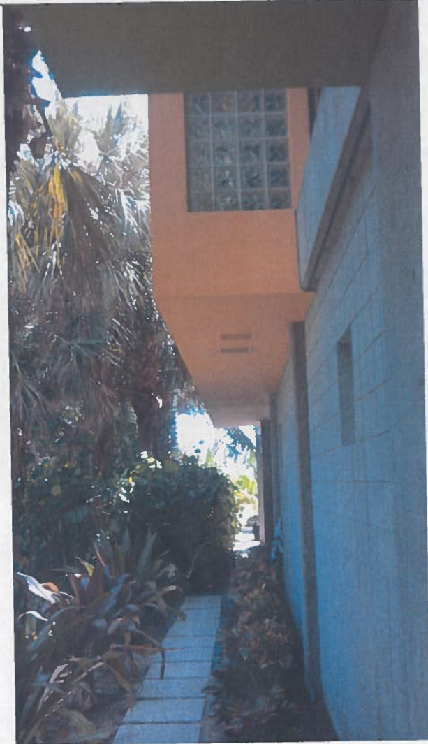
SIDE VIEW, SOUTH 6/24/2014
