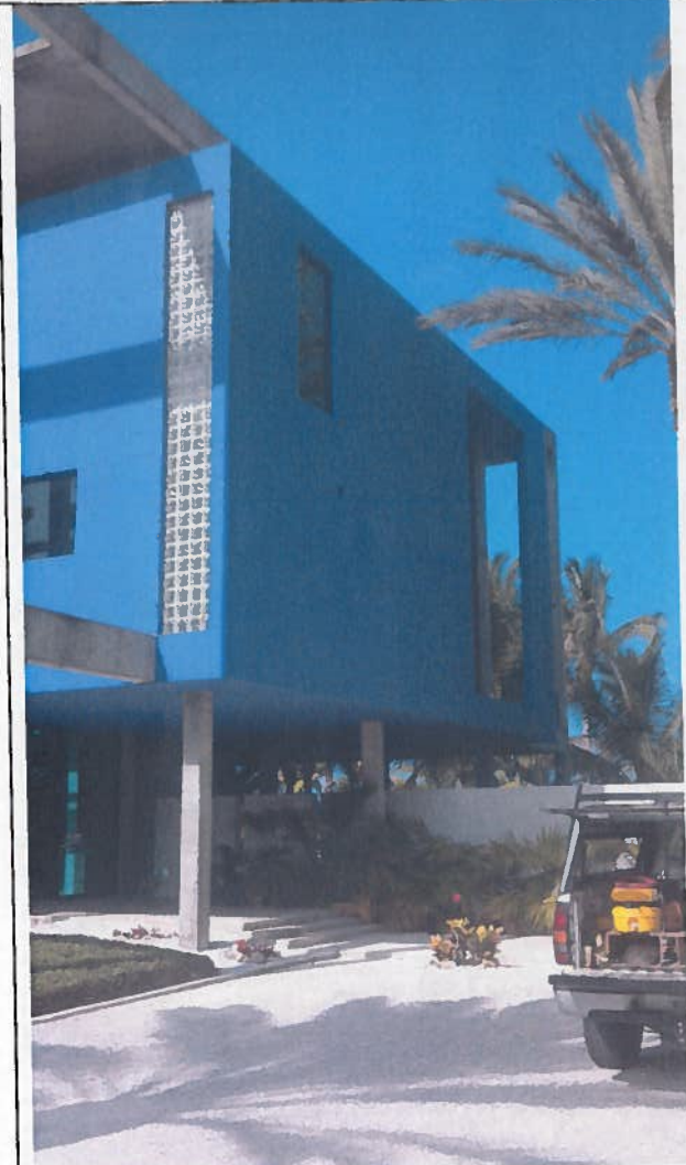
SIDE VIEW, NORTH 6/24/2014
