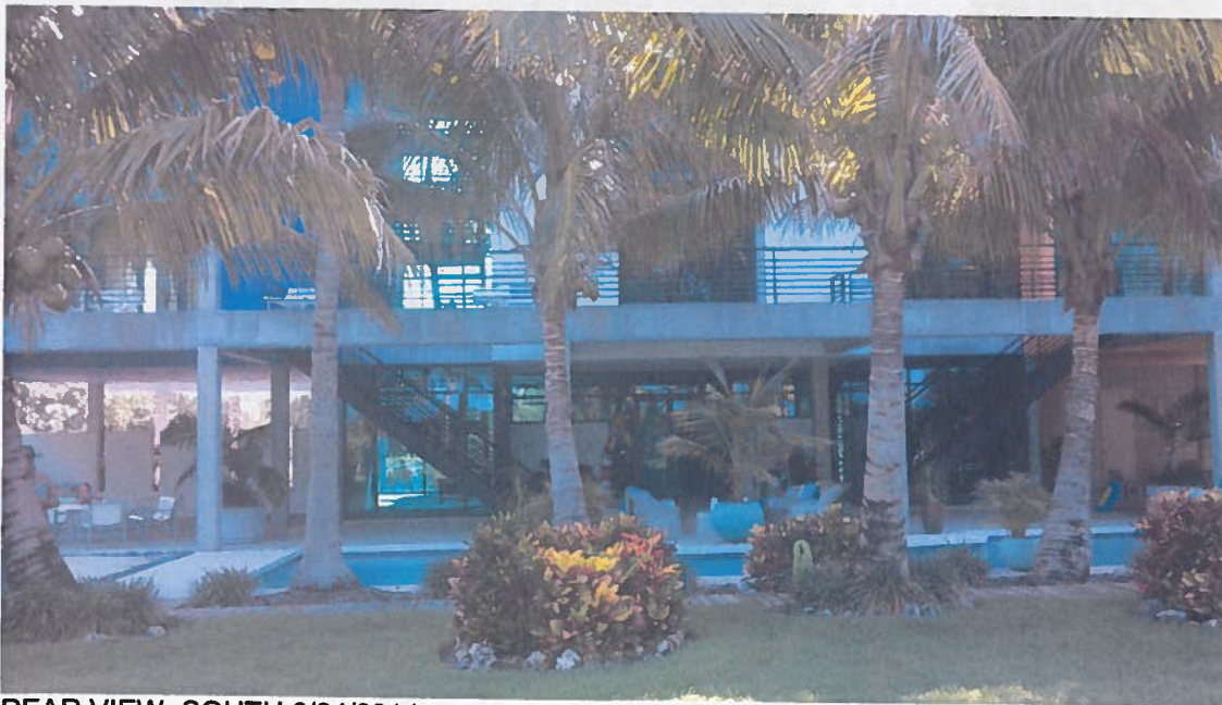
REAR VIEW, SOUTH 6/24/2014
