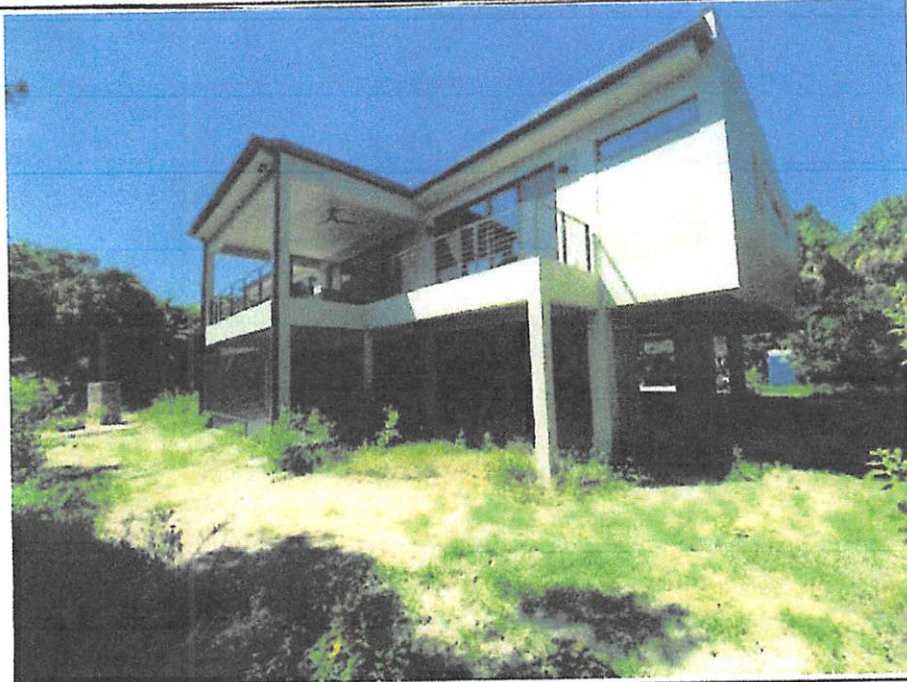
Photo Two Caption REAR PHOTO TAKEN ON OCTOBER 12, 2020
