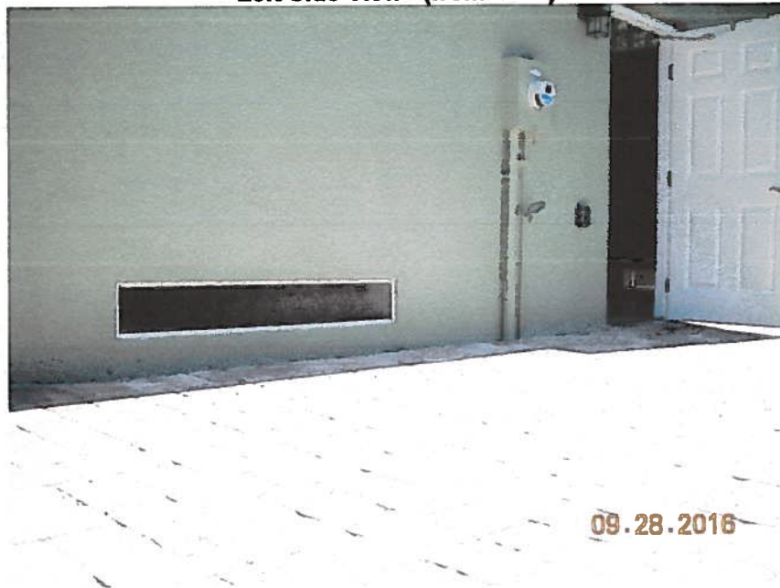
Typical Flood Vent
