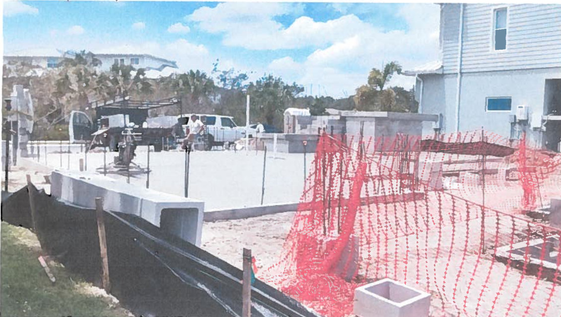
FIGURE 2: (05/05/15) REAR & RIGHT SIDE VIEW
