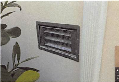
FLOOD VENT EXTERIOR VIEW 2/20/2025
