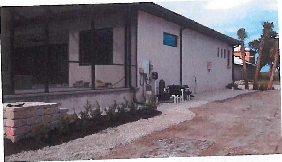
West Side of House:
