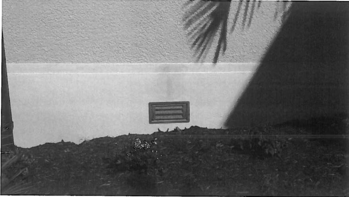
South Side of Garage one smart vent:
