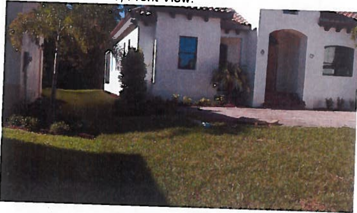
East Side of House, Front View:
