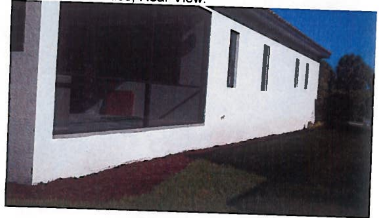
East Side of House, Rear View:
