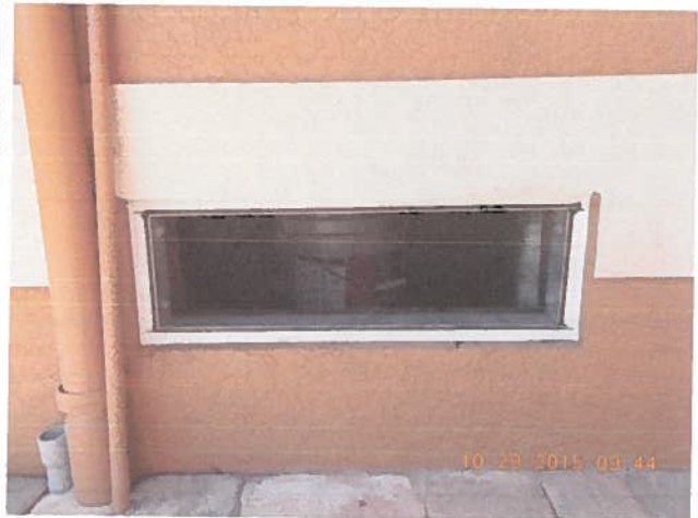
Typical Flood Vent
