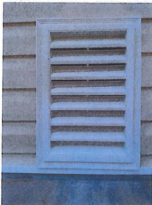
Two 10"x16" Flow Throughs in Storage Area Walls
