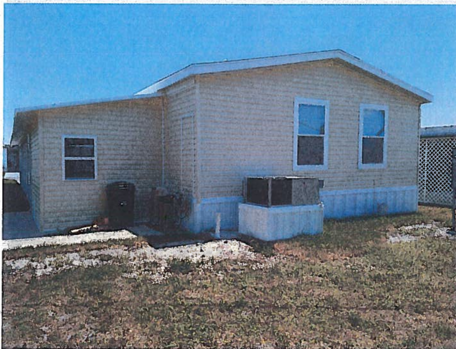
Photo Two Caption Rear View Date Taken 05/08/17 JOB# 15-1021
