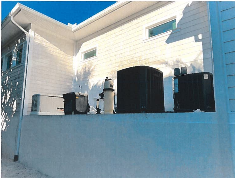
(01/17/2022) Elevated Platform with AC Units, Generator & Pool Equipment On Left Side of Structure = 11.4'.
