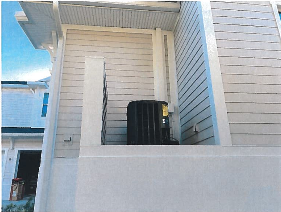
(01/17/2022) Elevated Platform with AC Units, Generator & Pool Equipment On Left Side of Structure = 11.4'.
