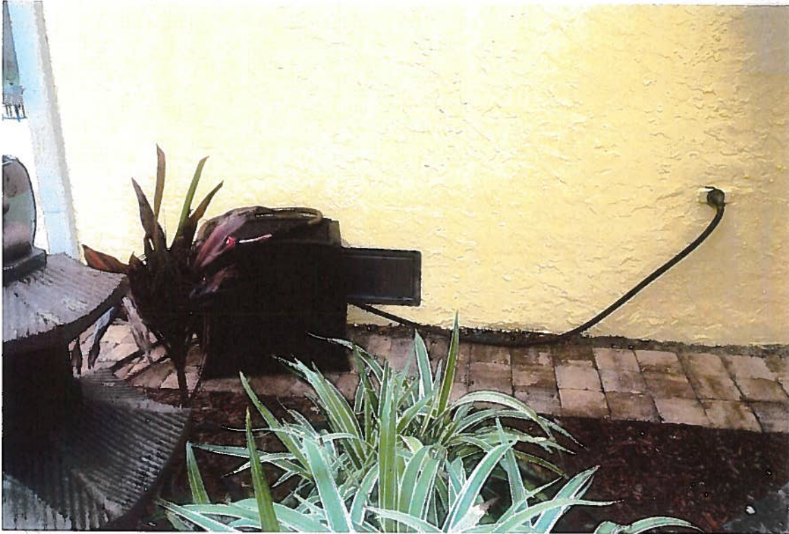
NORTH SIDE VIEW GARAGE
