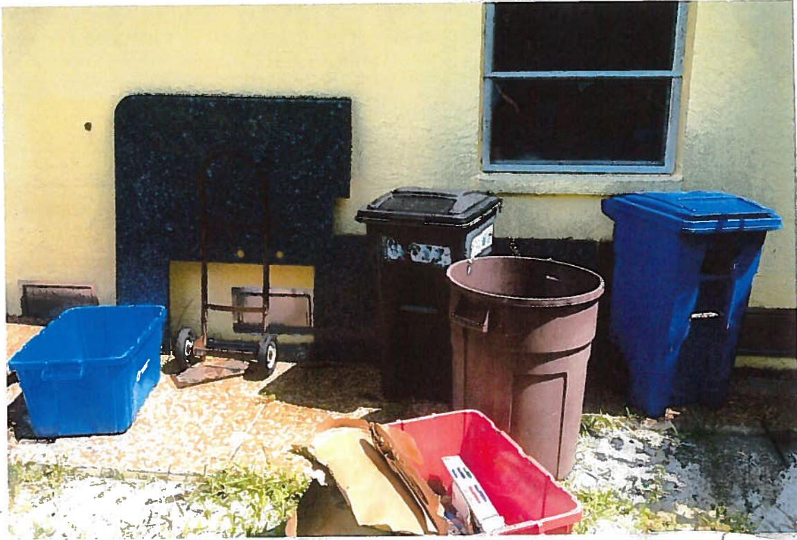
SOUTH SIDE VIEW GARAGE
