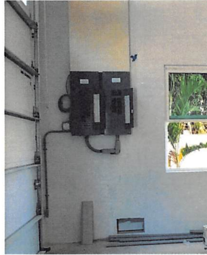
(10/27/2023) Hot Water Heater=10.3', Electric Panels=10.3', both in Garage
