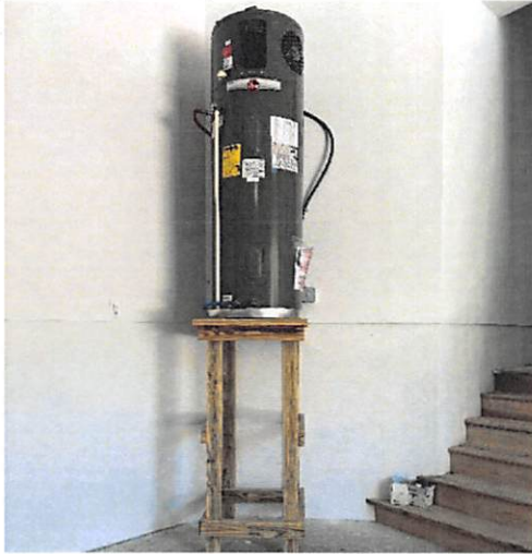
(10/27/2023) Hot Water Heater=10.3', Electric Panels=10.3', both in Garage
