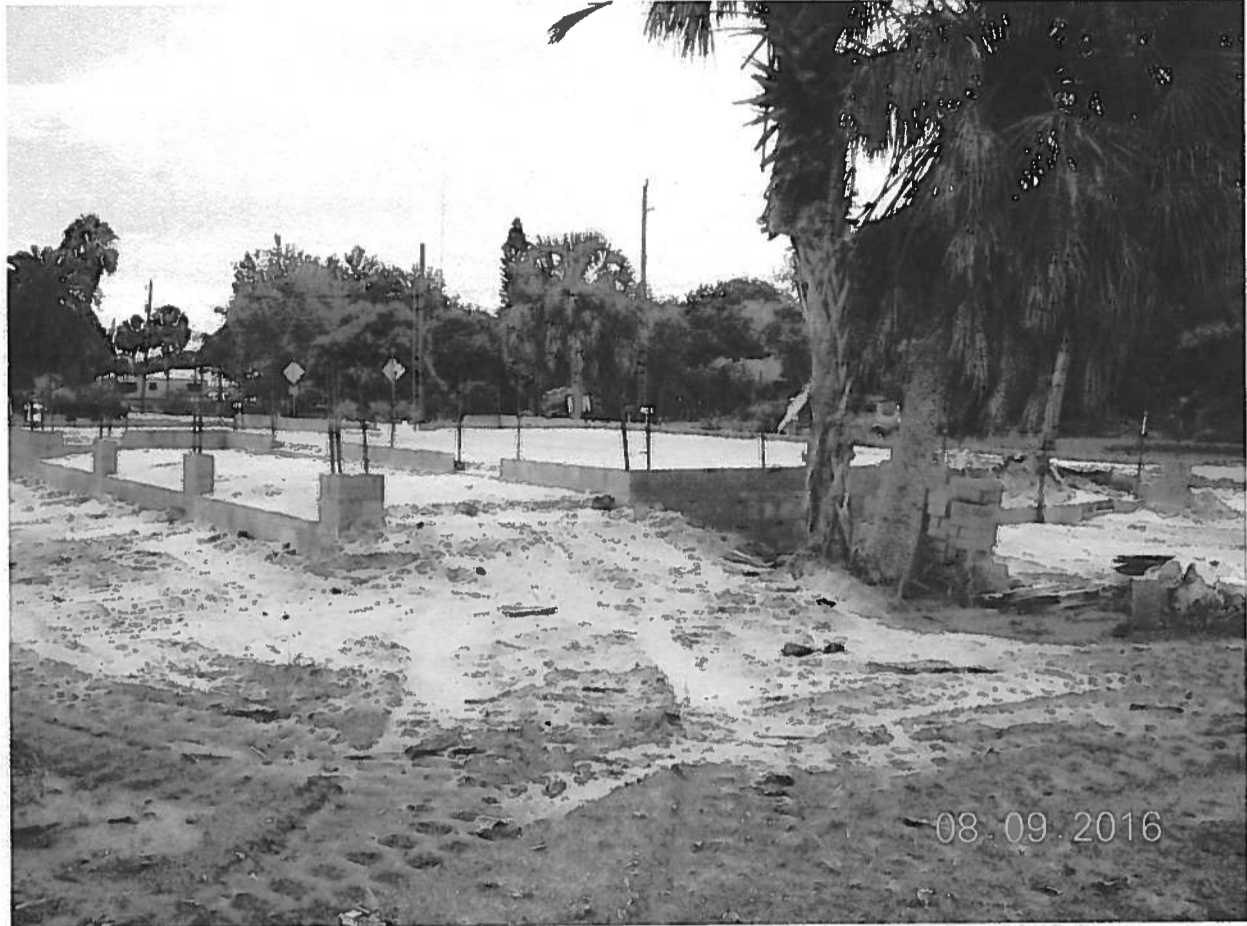
Rear View & Left Side View (from rear corner)
