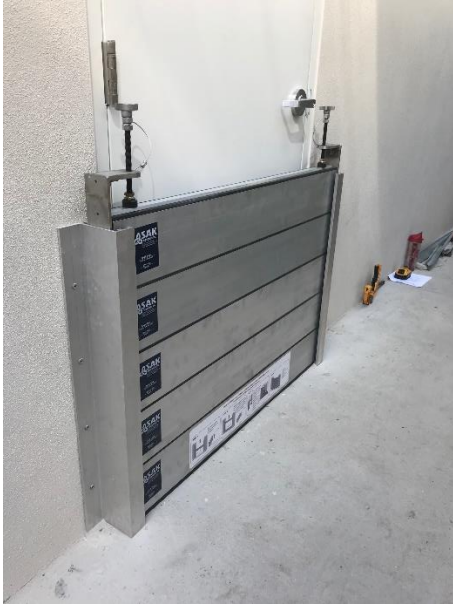
Rear Door Flood Panel Installation
