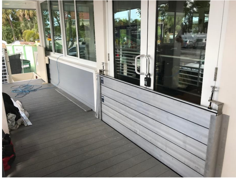
Front Door Flood Panel Installation
