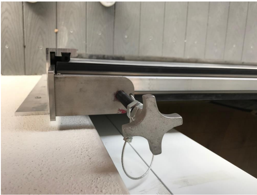
Front Door Flood Panel Wall & Panel Fastening Detail
