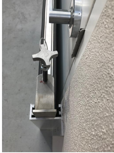
Rear Door Flood Panel Wall & Panel Fastening Detail
