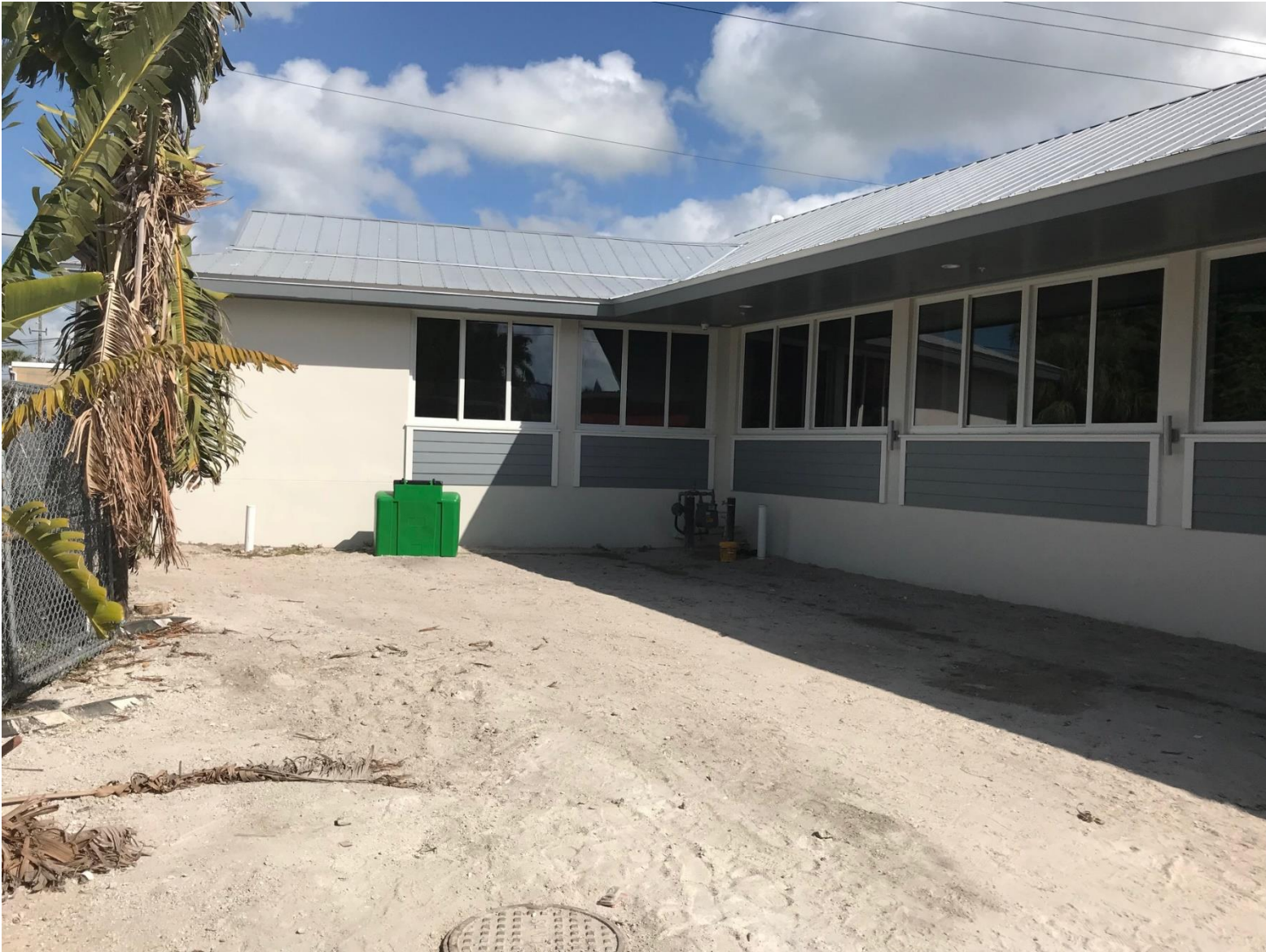
South Side / SW Corner Building Elevation – window sills 1' above FEMA BFE
