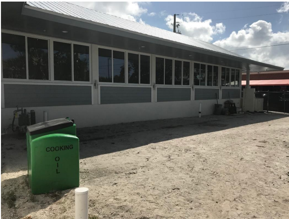
West Side Building Elevation – window sills 1' above FEMA BFE
