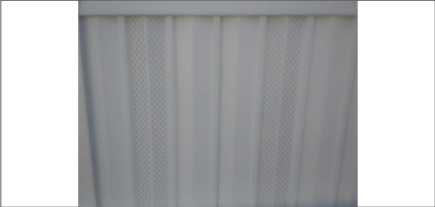
Photo 5 Caption Skirting under mobile home JOB# 19-1269 Date Taken 9/23/20
