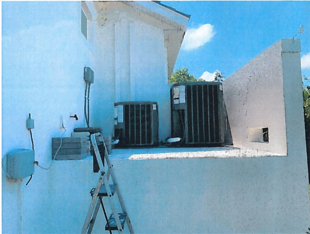
(05/06/2021) Elevated AC Units Outside of Structure
