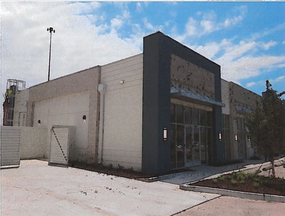
Photo Two Caption Side of Building under construction (Taken 05-05-2021)
