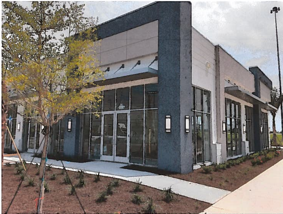
Photo Three Caption Rear of Building View (Taken 05-05-2021)
