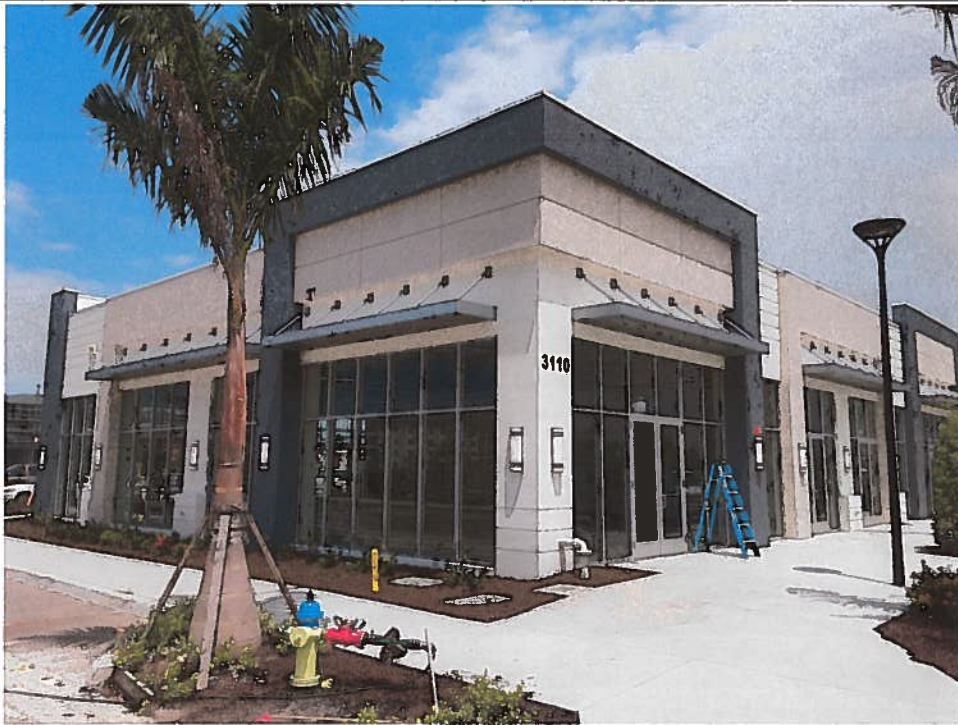
Photo One Caption Front of Building under construction (Taken 05-05-2021)
