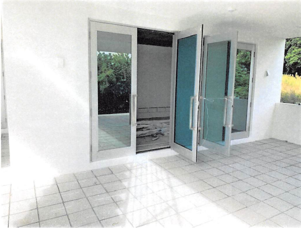
(10/23/2021) Pool Storage Area from Pool Deck
