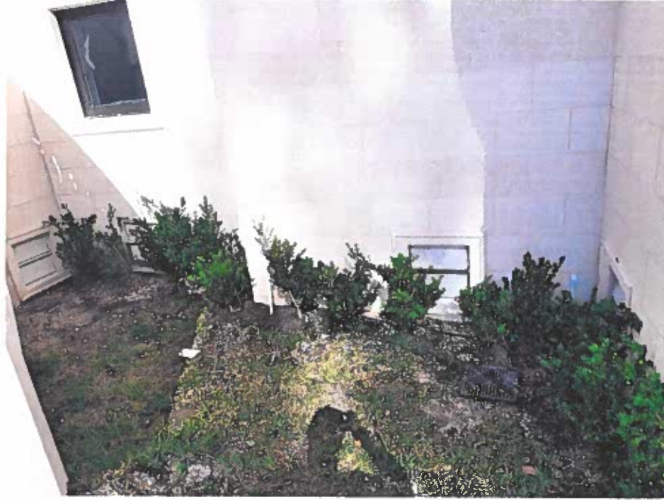
(02/13/2023) 3 Double Smart Vent Model #1540-521, 1 Single Smart Vent Model #1540-520 on Front-Right Side/Vestibule, Stairs & Storage 1
