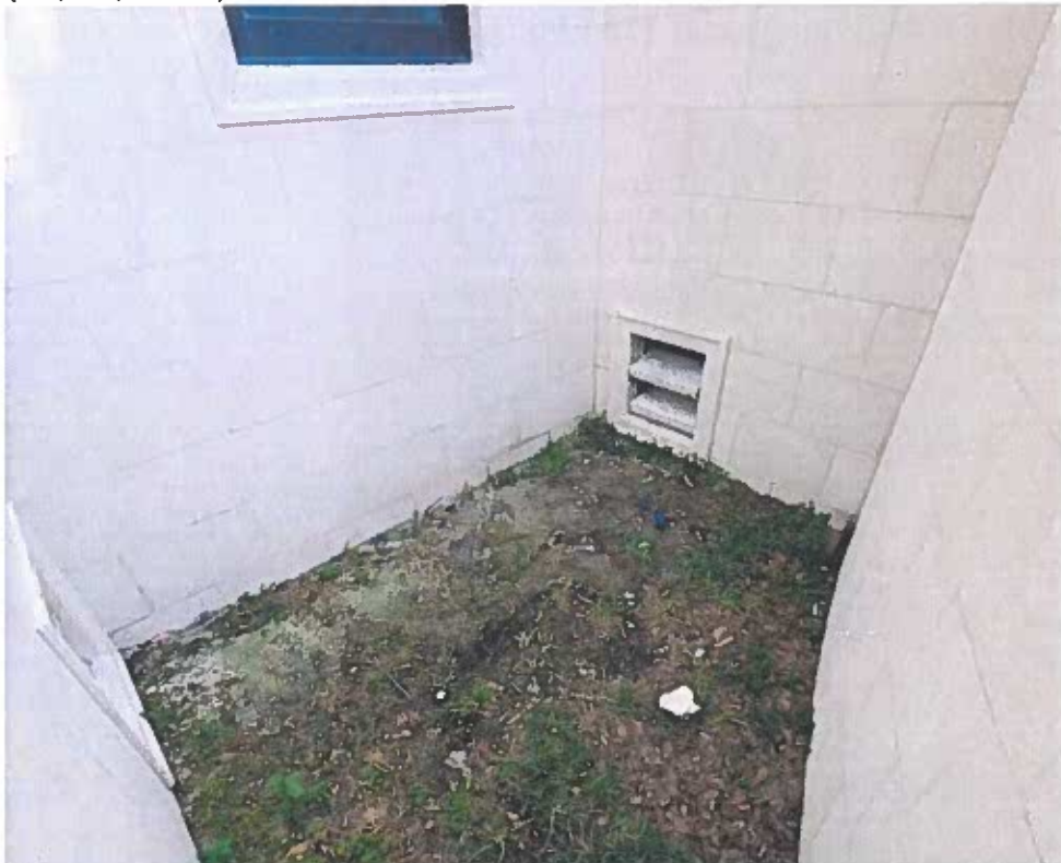
(02/13/2023) 2 Double Smart Vent Model #1540-521 on Front-Left Side/Storage 2
