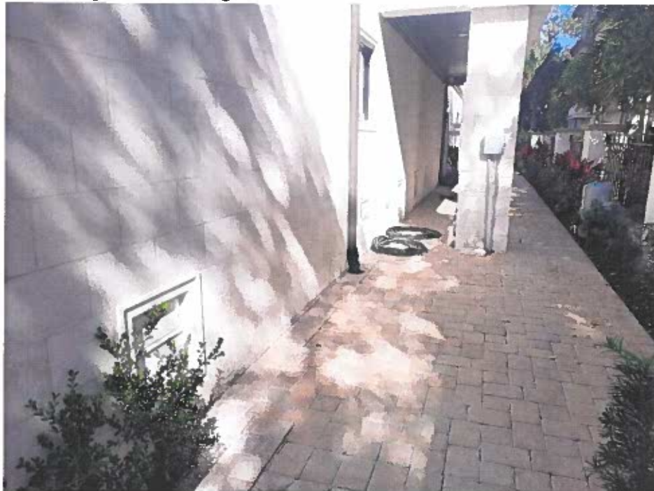
(02/13/2023) 5 Double Smart Vent Model #1540-521 on Right Side-Front Portion of Storage 1 & Storage 3
