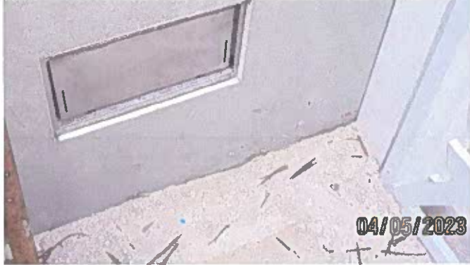
VENT AS LOCATED IN WEST WALL OF ENCLOSURE #1
