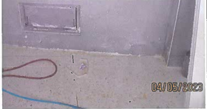
VENT AS LOCATED IN EAST WALL OF ENCLOSURE #1
