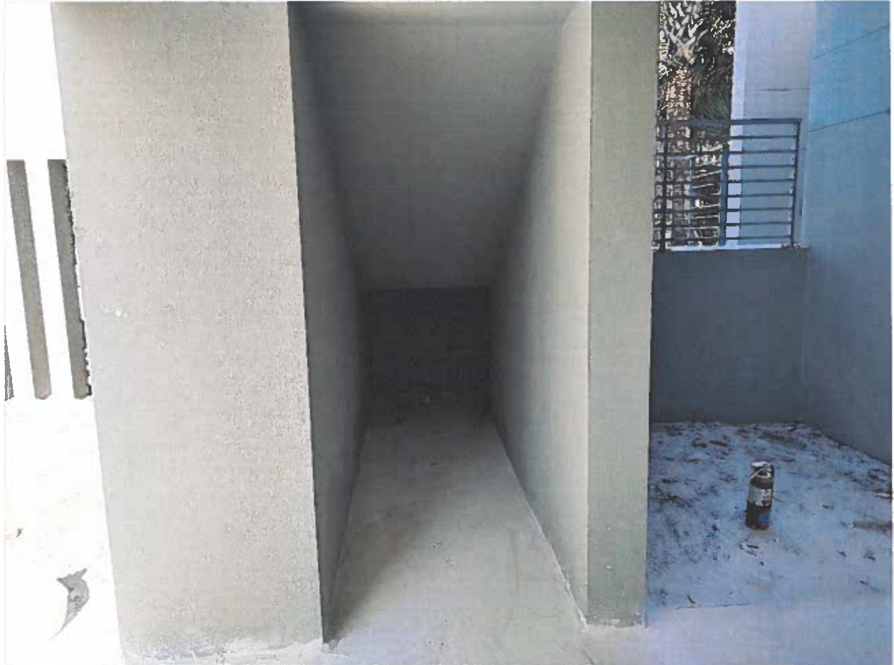
(05/05/2023) Opening/Entrance to Enclosed Area Under Stairs & Landing
