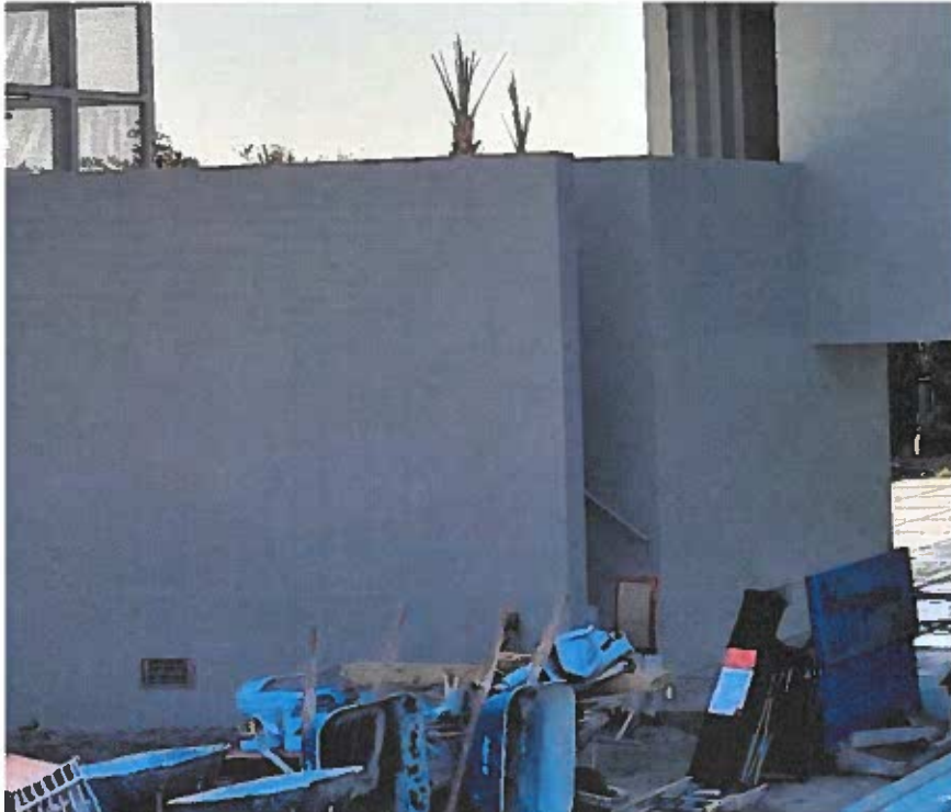
(05/05/2023) West Wall of North Structure Enclosure #1 1 Smart Vent
